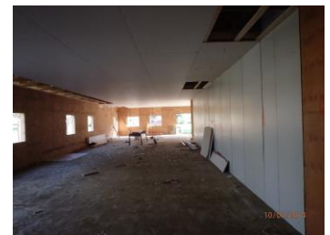
South side of east room.
