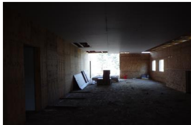
North side of east room.
